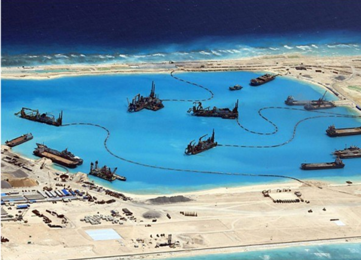
Construction at Kagitingan (Fiery Cross) Reef in the disputed Spratly Islands in the south China Sea by China. (Photo: EPA)
