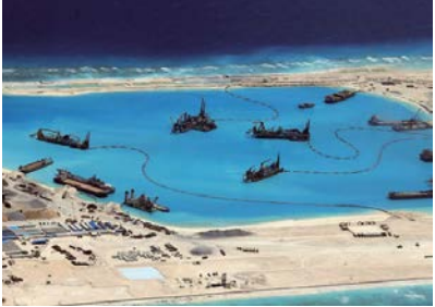
A photo provided by the Philippines last month shows construction by China at a reef in the disputed Spratly Islands in the South China Sea in February. (Photo/Armed Forces Of The Philippines)
