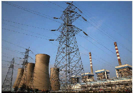
Cooling towers are pictured at a coal-fired power plant in Hubei, east China's Jiangsu province, June 20, 2016. (Photo/ImagineChina)
