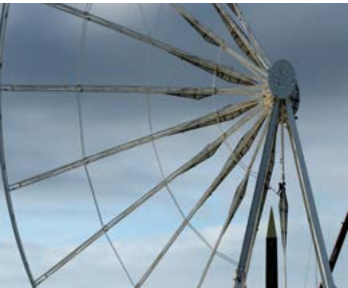
A worker climbs up the giant Ferris wheel of the Place de la Concorde as it is being rebuilt before the Christmas season in Paris
