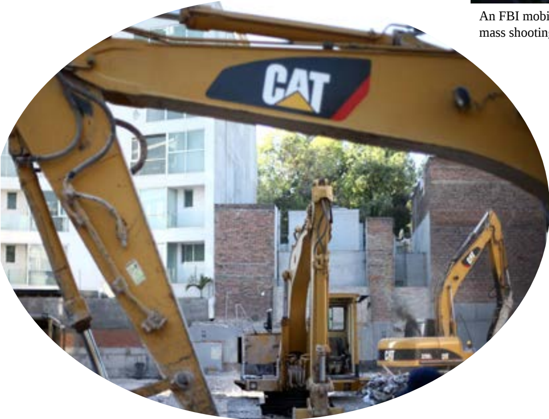
Diggers are pictured at a site where a building was demolished and where a memorial park in honor of the victims of the September 19 earthquake will be built, in the La Condesa neighborhood in Mexico City MEXICO-QUAKE/
