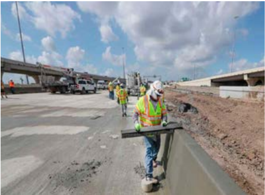
The construction area for U.S. 290 project near Fairbanks North Houston Road Thursday, June 28, 2018, in Houston
