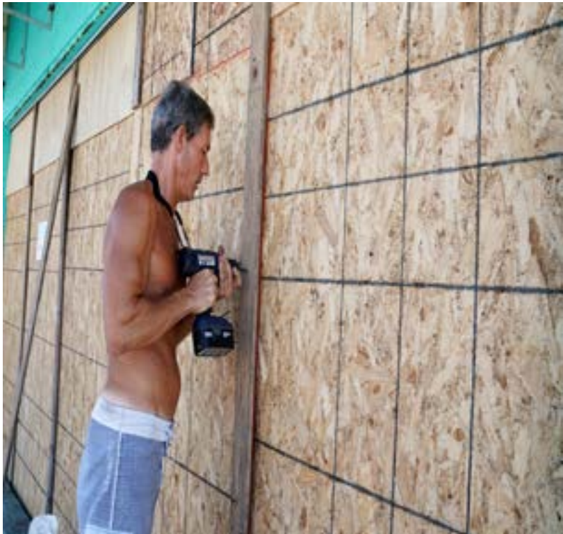
A man puts plywood up on the windows of his store before Hurricane Florence comes ashore in Wrightsville Beach
