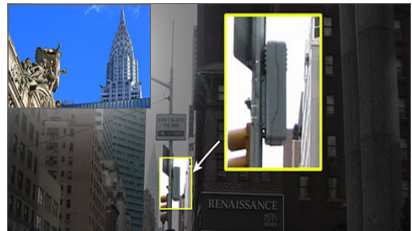
A 5G box attached to a lamp pole at the corner of East 57th Street, close to Times Square in New York City.
