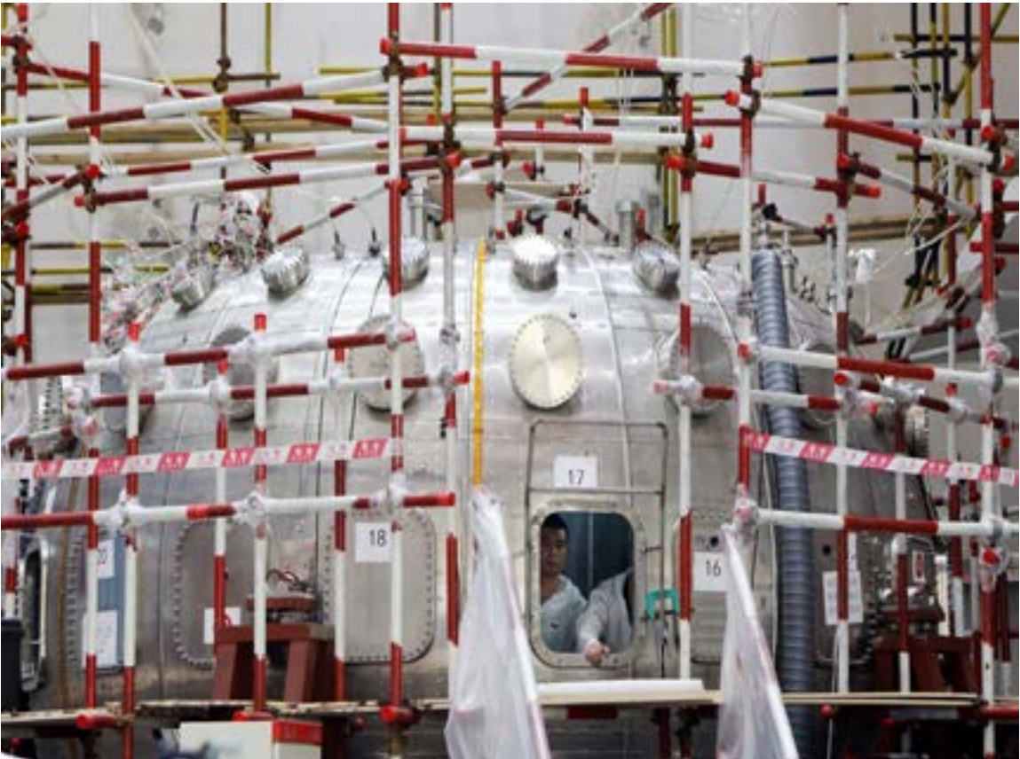
Men work inside a HL-2M Tokamak nuclear fusion reactor under construction in Chengdu
