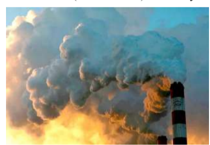
Smoke and steam billow from Belchatow Power Station, Europe's largest coal-fired power plant, near Belchatow, Poland. Picture taken November 28, 2018. REUTERS/Kacper Pempel/File Photo
