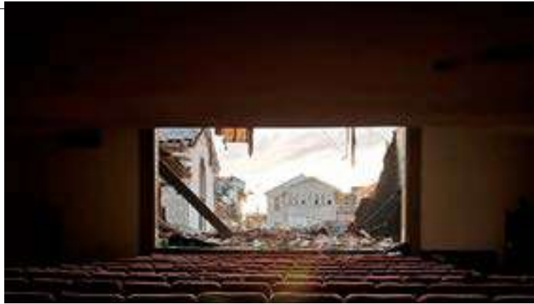
Debris are picture from a cinema after tornadoes ripped through several U.S. states in Mayfield, Kentucky. Shawn Triplett/via REUTERS
